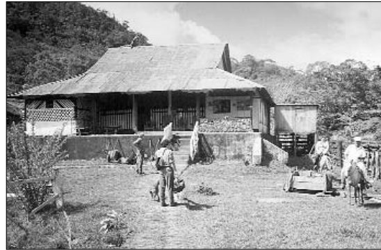
The main multi-purpose building at Los Chavalitos.
