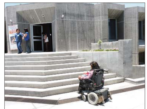
Wheelchair access remains a big problem in Peru, even in public buildings. This guest speaker in Chimbote confronted these stairs at the hospital auditorium where our disability seminar was held. Participants helped carry her up.
