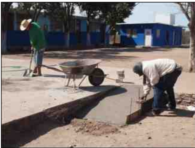
To make the play-area and classroom wheelchair accessible, the rehab team and school staff organized a volunteer town project to build the necessary ramps.
